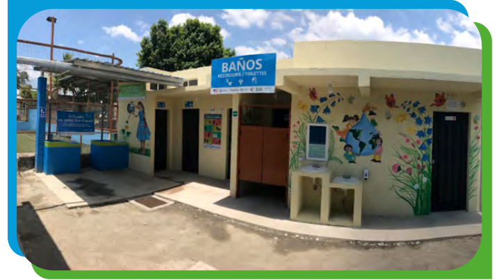
Sanitary module at the Carlos Roberto Reina Temporary Rest Center, in Trojes.
