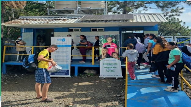
Semi-permanent module with attention to women and children, installed at the Machuca assistance point.
